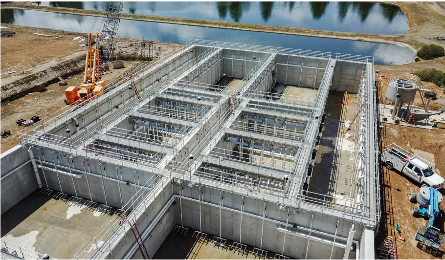
The ClarAtor clarifier equipment is installed into concrete tankage, utilizing common-wall aeration basin construction, helping to lower capital and construction costs.
